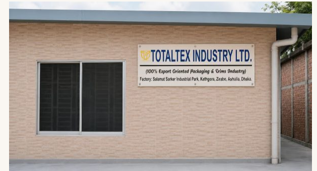
THE ZIRABO FACILITY, ASHULIA
